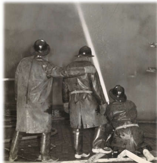
1946 - Downtown Stillwater Fire - Chestnut Street
