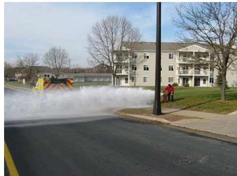
Annual Hydrant Flushing
