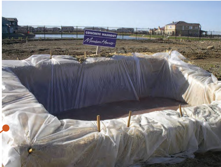
Photo 1: Well-maintained and labeled concrete truck washout
