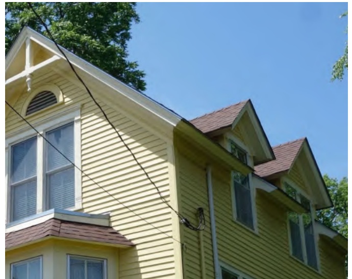
Dormers provide additional light, air and headroom to attic spaces. Dormers project through a sloping roof, and usually repeat the same roof form as the main roof.
