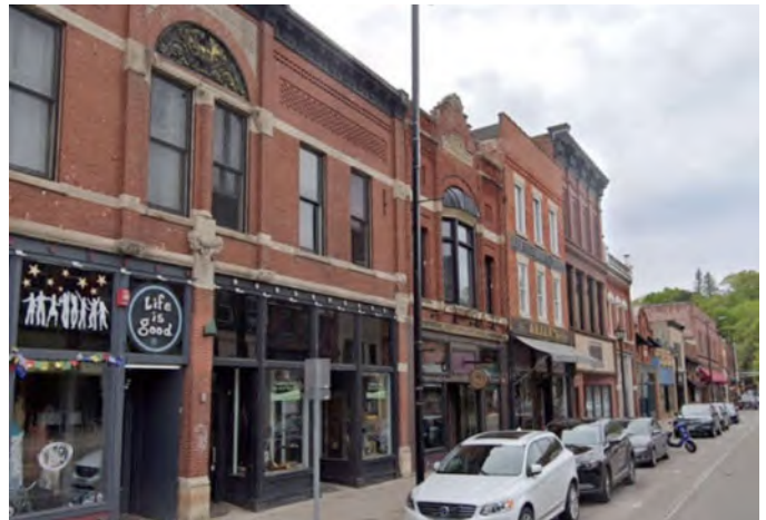
The top photo shows the east side of S. Main Street, looking south, in 1974. Below, façade rehabilitation, including brick conservation and removal of large signs and metal cladding, has transformed the appearance of this block. MNHS
