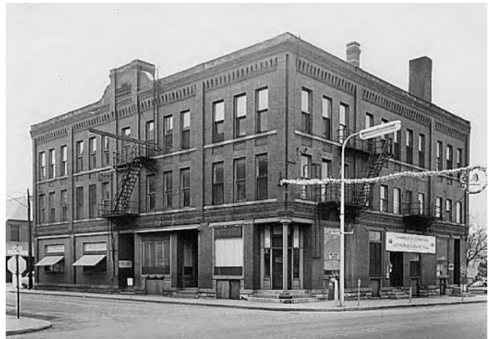
Lumbermen's Exchange, 101 S. Water Street (1890). MNHS
