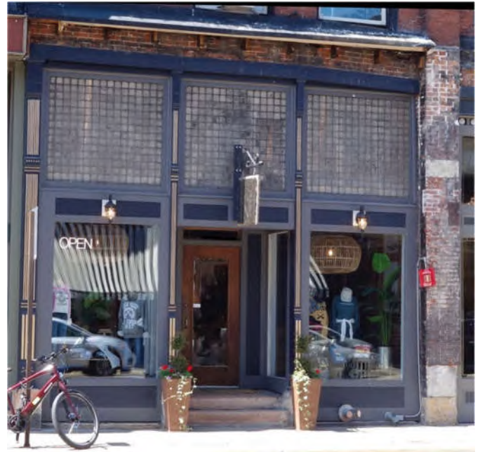
Restored storefront, ca. 1884, at 216 S. Main Street.
