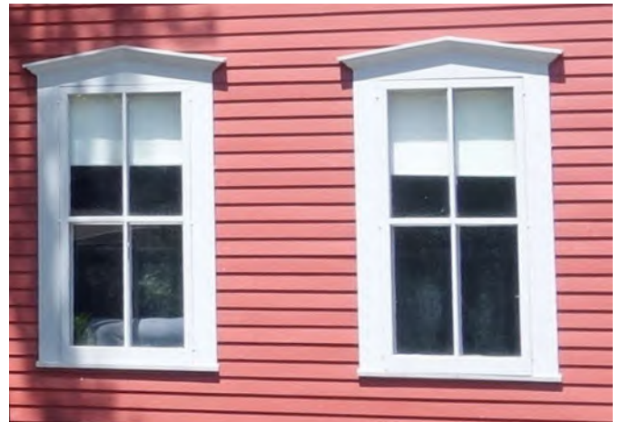
Parts of a Greek Revival style window shown with 2-over-2, double-hung sash
