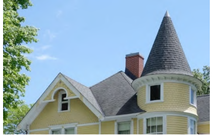
The shape, texture, and color of the roof are key design features of the historic building. New dormers and other additions to the roof must be carefully designed. In Stillwater, wood shingles were used to roof the earliest houses, and asphalt shingles became standard in the early 20th-century. Gordon and Ida Welshons House, 117 Burlington Street (1887).
