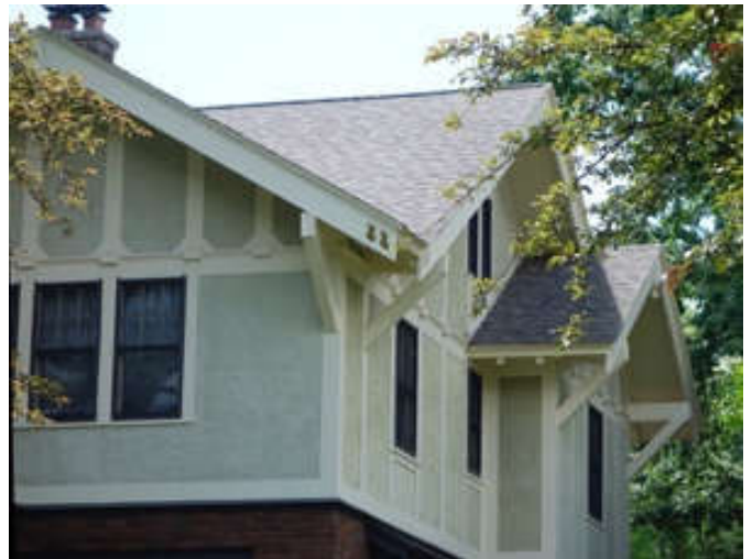
Decorated bargeboards, knee brackets, and paneling decorate the eaves and upper story of this Craftsman style house.
