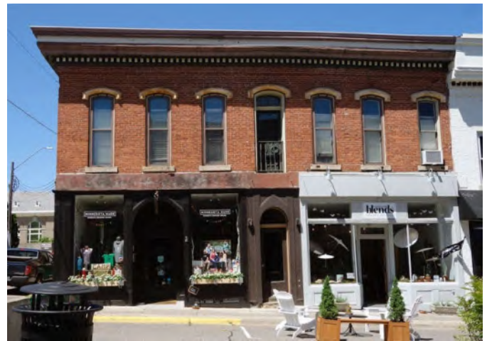
This Italianate style business block at 220-224 E. Chestnut Street dates from before 1884 and features a lancet-arched central entry, deep overhanging eaves, and stone hood molds above the slender double-hung windows. The storefronts have central entries flanked by large display windows.
