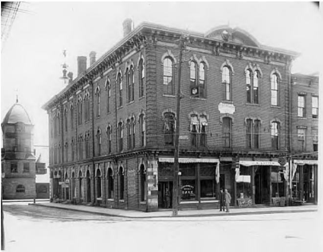
The Hersey & Staples Block in 1914; the Union Depot is at rear (both razed). MNHS
