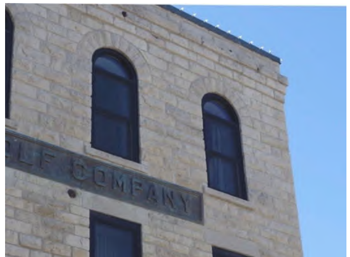
Above: locally quarried limestone and many types of brick, including locally burned yellow brick, are among Stillwater's distinctive early building materials.
