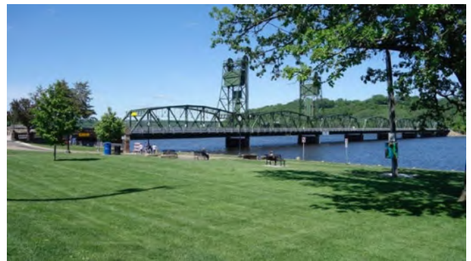
Stillwater Lift Bridge and Lowell Park, 2021.
