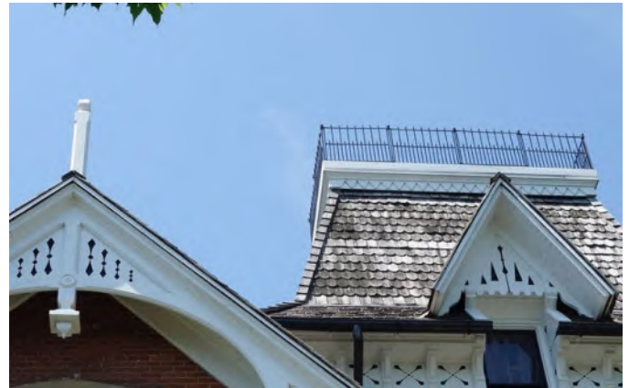
Captain Austin Jenks House, 504 S. 5th Street (1871, NRHP).
