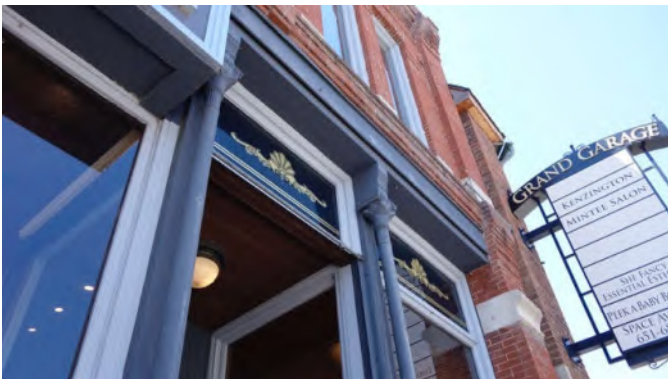
Restored storefront at 330 S. Main Street; building dates from ca. 1885.
