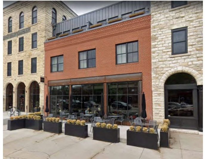
At the Lora Hotel at 403 S. Main Street, the façade of the two-story red brick building (which dates from the 1980s) was restored and features new display windows. A new penthouse above has simple exterior cladding and window openings.
