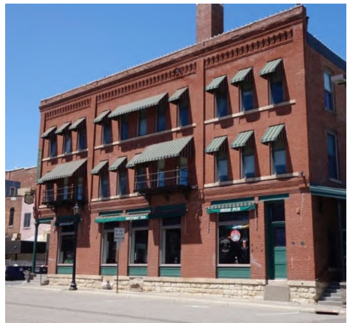
Awnings at the Lumbermen's Exchange, 101 S. Water Street (1890).
