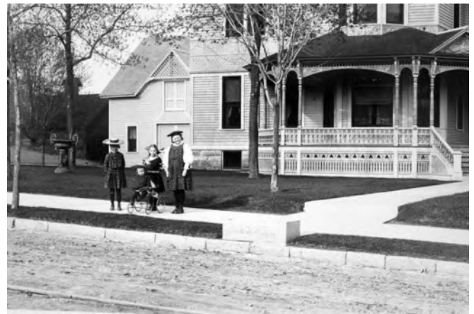
Photographs, maps, and other building records at the Washington County Historical Society, Stillwater Public Library, and Minnesota Historical Society document past changes to Stillwater's historic houses. The Hospes House at 4th and Mulberry Streets is shown in 1921. MNHS/Runk
