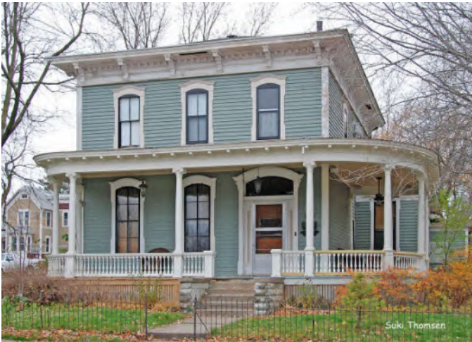
John G. and Johanna Nelson House, 604 N. 4th Street (1874). The curved porch dates from ca. 1905. Suki Thomsen photo
