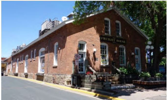
Chicago, Milwaukee & St. Paul Depot and Freight House (1883, NRHP). Multi-paned, segmental-arched windows and a deep limestone foundation are notable features.
