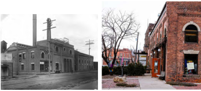
At left, the NSP Substation (ca. 1904) in ca. 1920; at right, the Brick Alley, 432 S. Main Street, in 2019. (WCHS/Runk)
