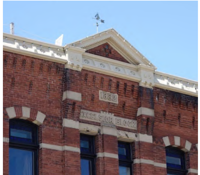
Excelsior Block (1882) at 118-126 N. Main Street features a corbeled brick cornice and stone date and name plaques.
