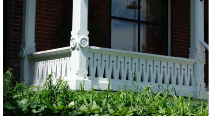
The details of this baluster and rosette-trimmed, chamfered porch post should be kept intact, if possible. Wood trim can be treated with preservatives and paint. Any trim that must be removed should be saved as used as a pattern for replacement.
