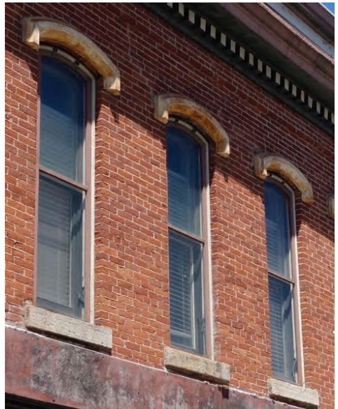
222 – 224 E. Chestnut Street, ca. 1882. Molded stone lintels and stone sills frame slender windows with double-hung sash.
