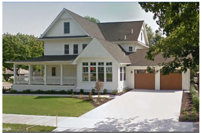
New residential construction at 207 E. Pine Street (2017).
