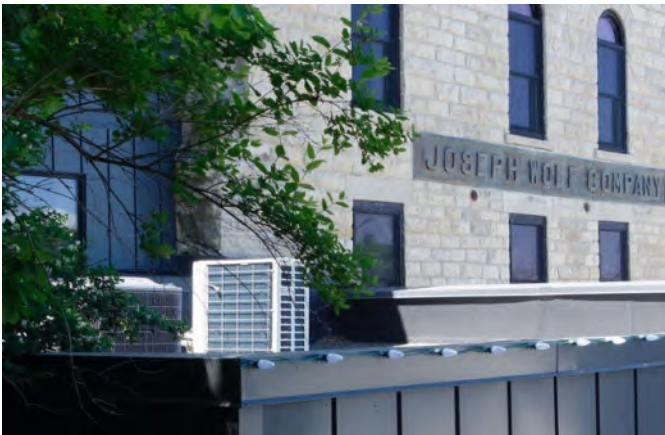
Rooftop equipment should be set back as far as possible.
