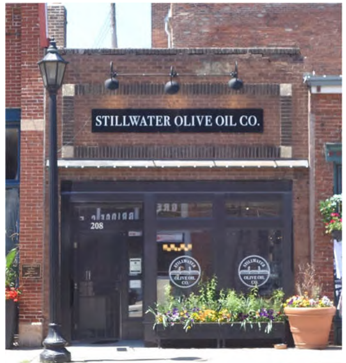
Restored storefront at 208 S. Main Street. The building dates from ca. 1904.
