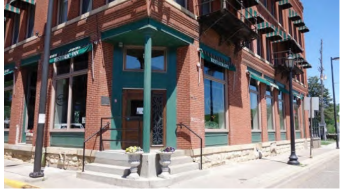
Lumbermen's Exchange, 101 S. Water Street (1890). MNHS
