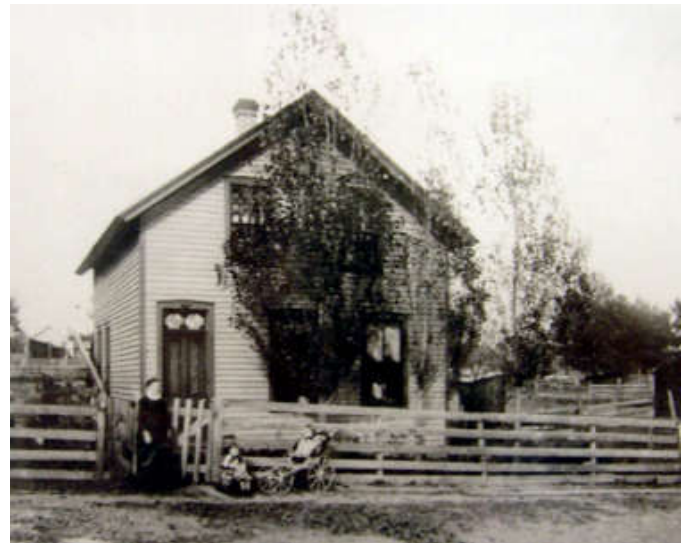
A simple vernacular house at 408 W. Maple Street (ca. 1875). WCHS
